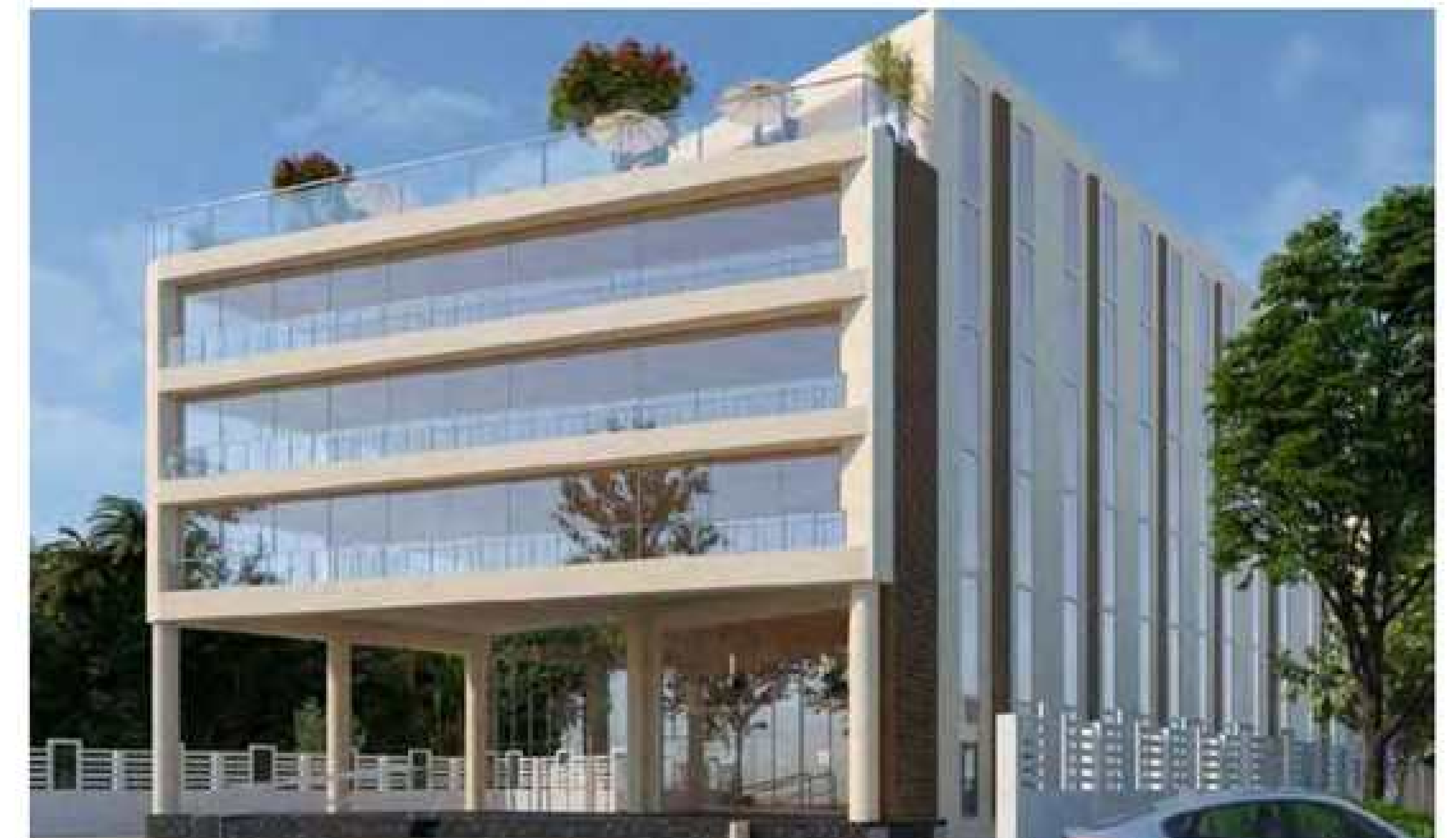
ECHO POINT PLAZA, COIMBATORE
