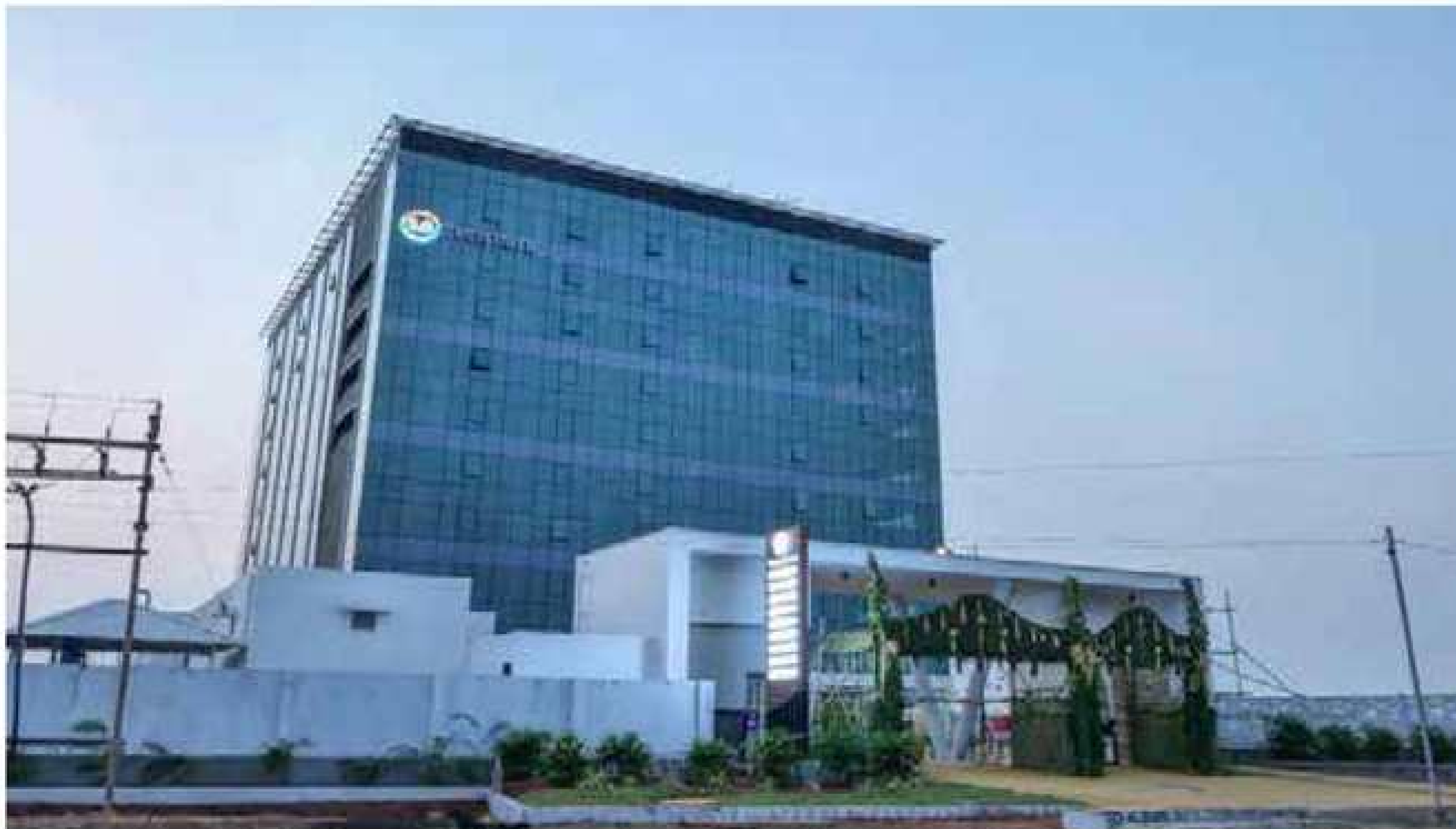
SVB TECH PARK, COIMBATORE
