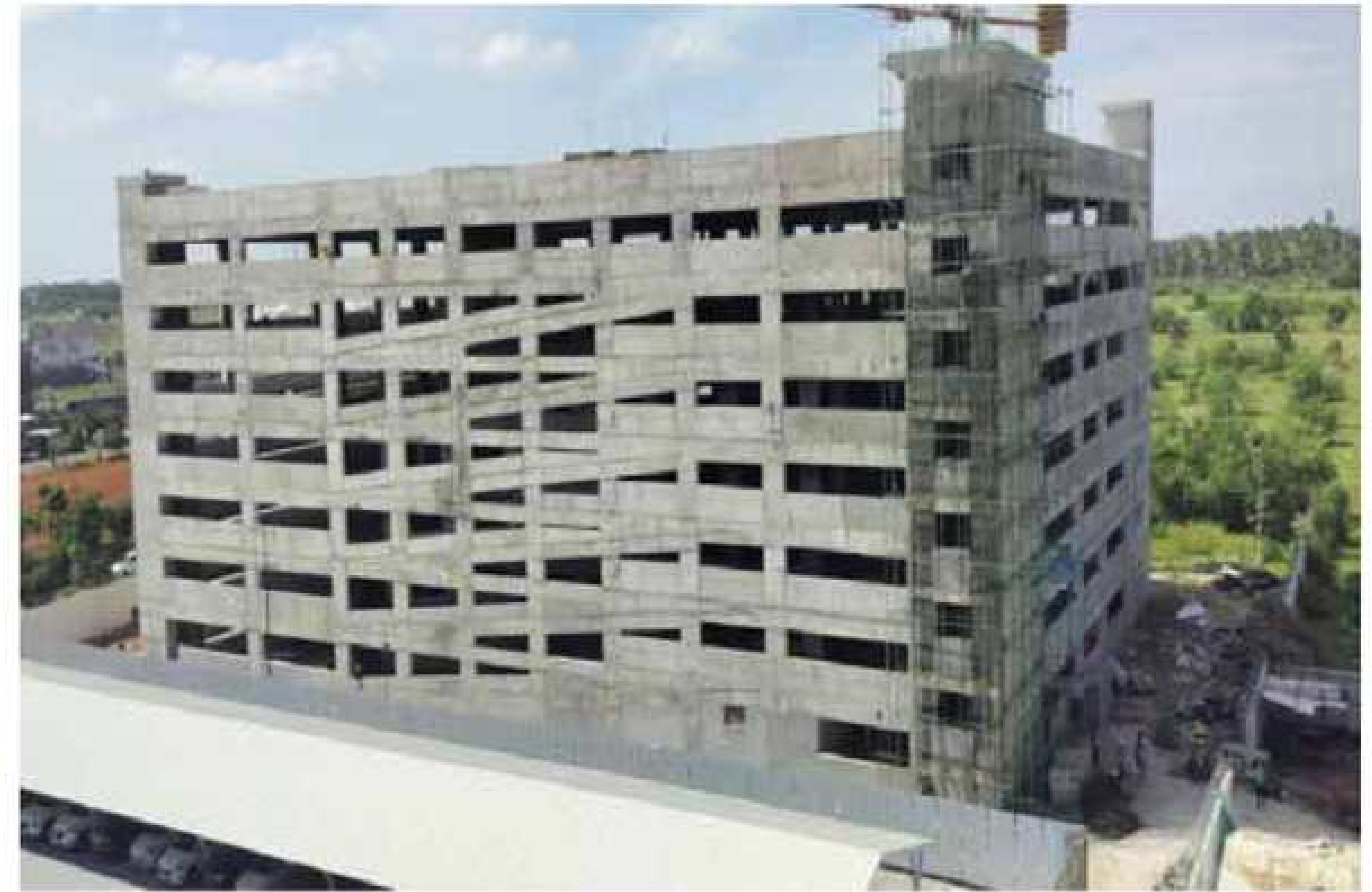
SVB Multi Level Car Parking (MLCP), COIMBATORE
