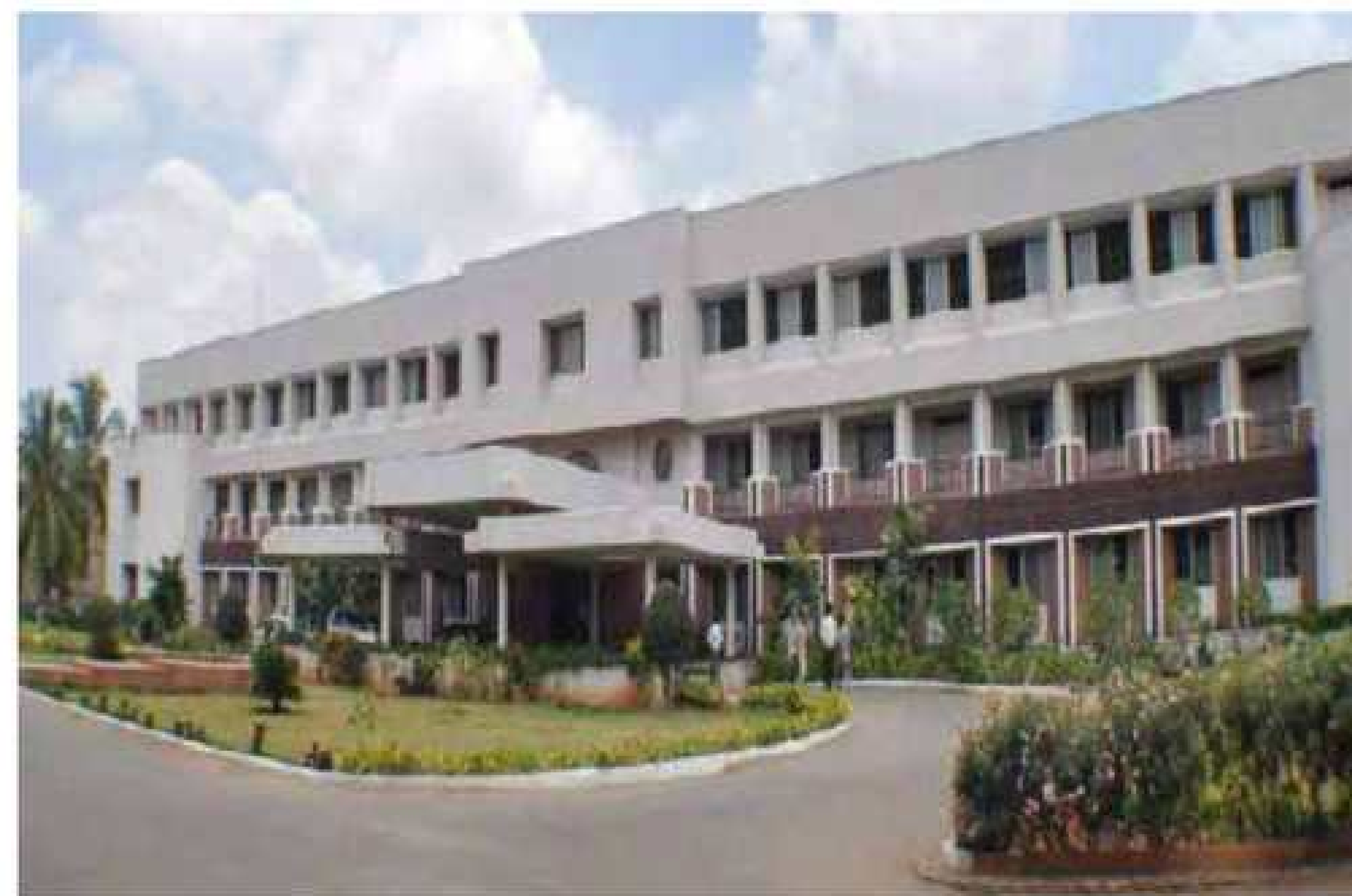
SRI RAMAKRISHNA ENGINEERING COLLEGE, COIMBATORE
