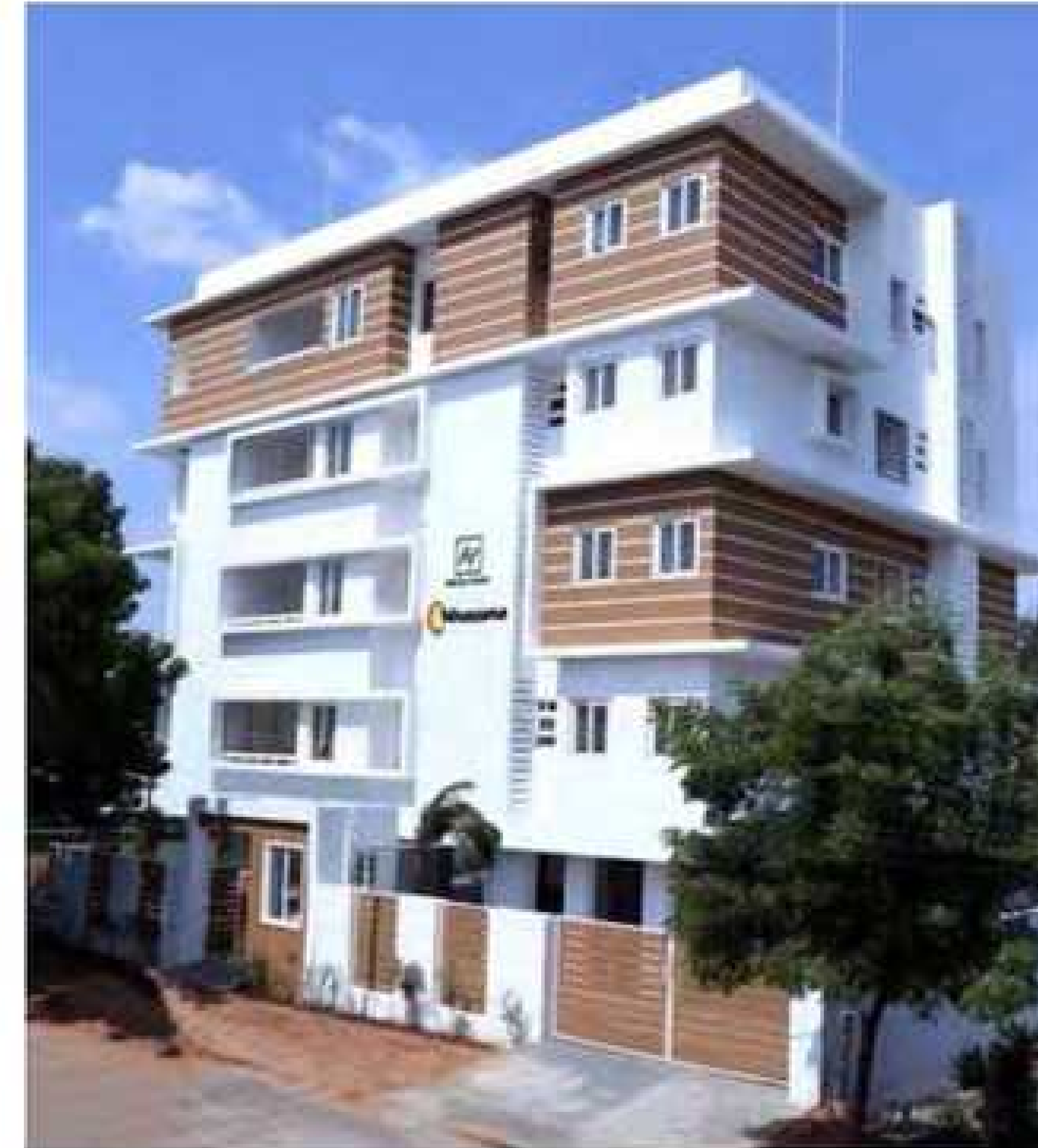
NIVASANA APARTMENTS, COIMBATORE
